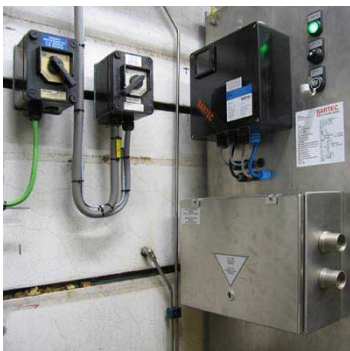
A Vortec cooler is used to cool the cabinet < 30 degrees Celsius
