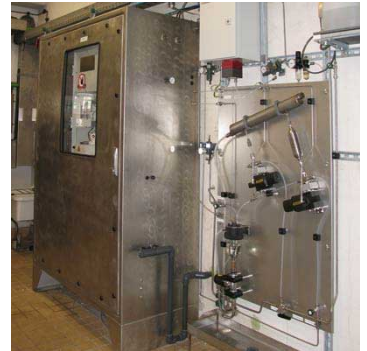
The Ex p cabinet complete with external sample conditioning
