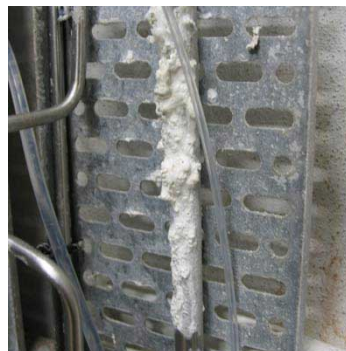
The sample contains components that "sweat out" pipe connections
