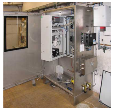
Good access for maintenance is "a must".
