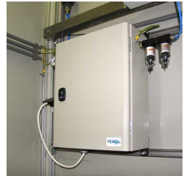
Pressure Swing Absorption is used to remove CO 2 from instrument air
