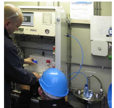
Commissioning and start up of the TOC-analyser by ODS engineers
